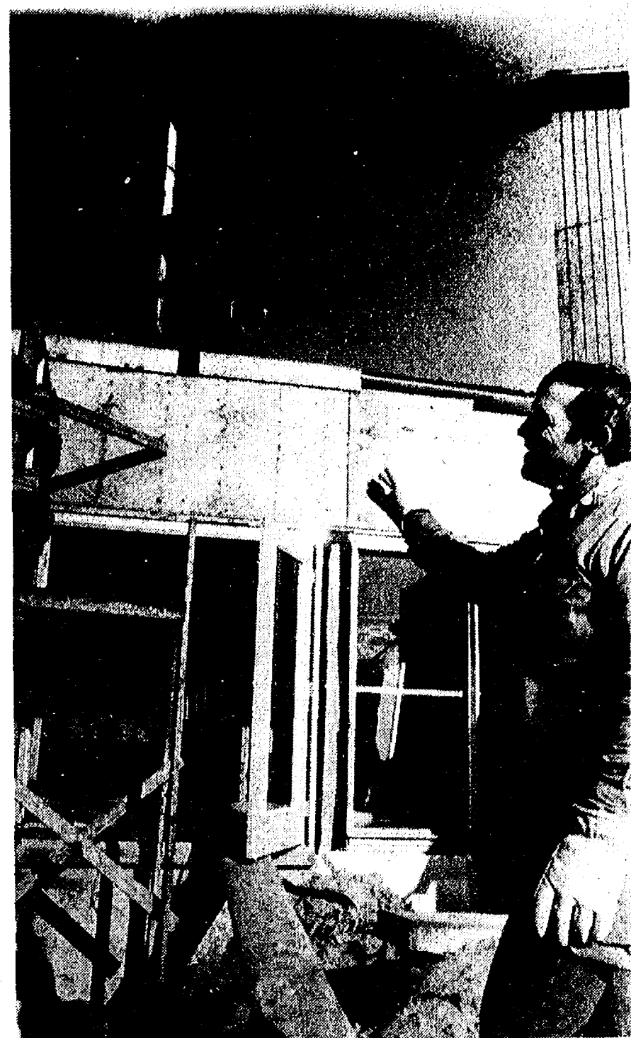
CHELSEA FREE METHODIST CHURCH , located on Werker Rd., is surveyed by co-ordinator John Eisenbeiser. Progressing on schedule, it is hoped that the new facility will be ready for occupancy by late December or early January. The solar facility, designed by an architectural firm from Chicago, is being constructed by a local contractor and is one of the only church buildings of its kind to be erected in the state. Meari Bradley serves as pastor of the church.
